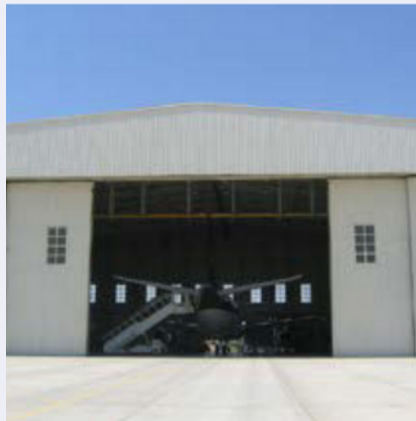
AIRCRAFT HANGAR DOORS
