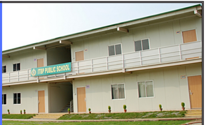
MULTI STOREY SCHOOL
