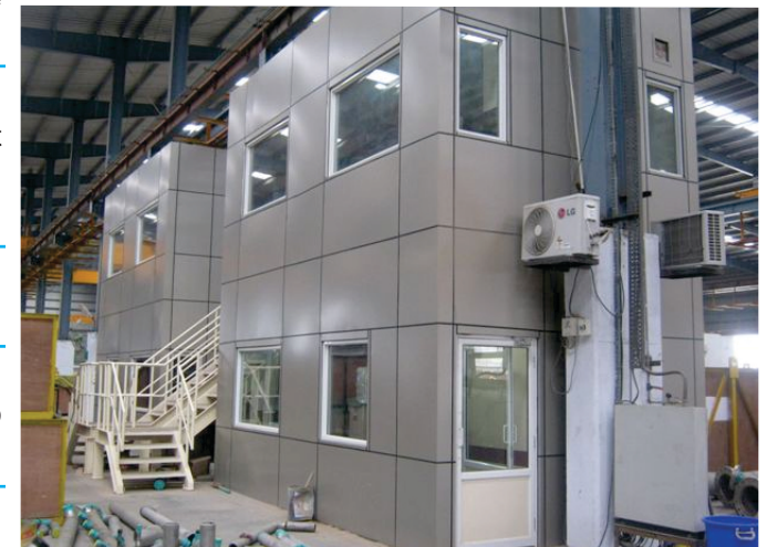
Double Story Control Rooms
