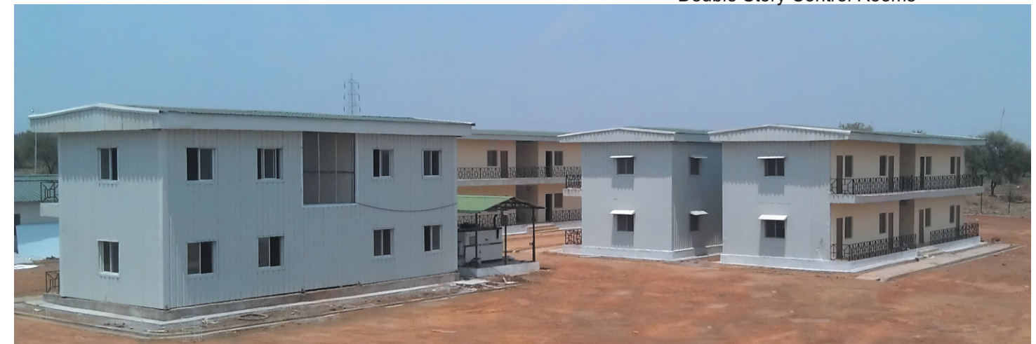
Double Story Township
